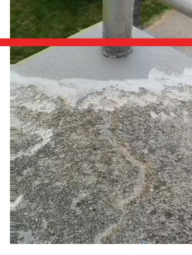
A wooden mold with Belzona 9411 (Release Agent) was used to achieve the correct dimensions. Then, a trowel was used to achieve a smooth finish.
